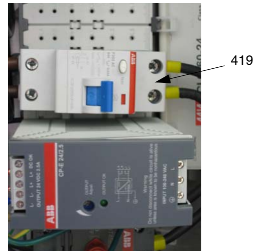
FIG. 32: Ground Fault Circuit Interrupter
